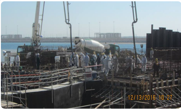
Deck Slab Pouring For Seawater Intake Structure
