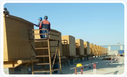
Installation of steel sheet
