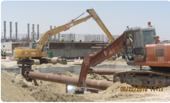
Excavation for Seawater Intake Structure
