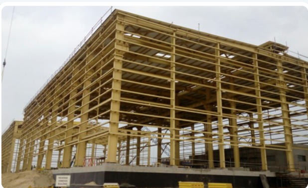
Construction Phases for RO Building Hot Rolled Steel Structure
