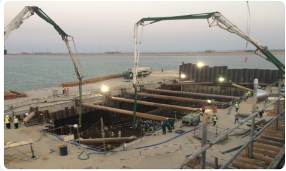
Concrete Pouring for SWI Base Slab
