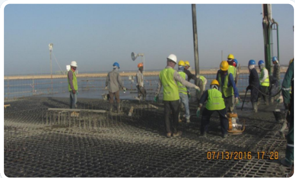
Concrete Pouring of Electrical Building Roof Slab
