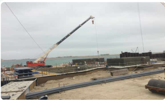
Seawater Intake Structure with GRP Gratings
