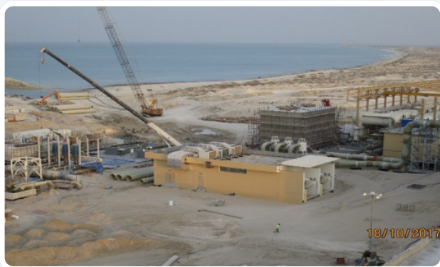
Reverse Osmosis Building
