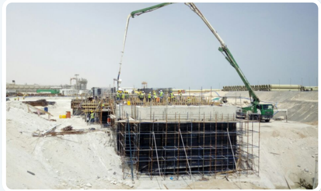
Construction Phases in Sea water Intake Structure
